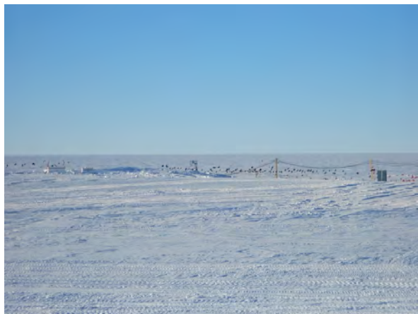
Fig 1. View of the (buried) arch at the end of the 2012-2013 field season. The power poles on the right-hand side of the photo lead back towards camp. The ventilation conduit in the center of the photo marks the start of the drilling arch, which then runs 100-feet to the left. The core handling arch runs to the right of the conduit for 84-feet. Photo: Don Voigt.
