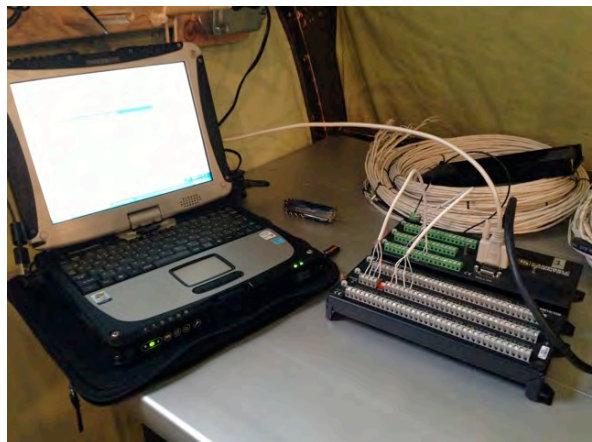
Fig 13. Programming and testing a logger. Photo: John Fegyveresi.
