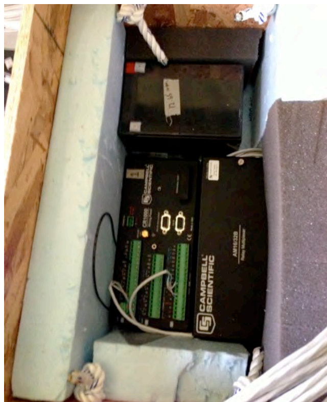
Fig 12. Building a logger housing-box. Photo: John Fegyveresi.
