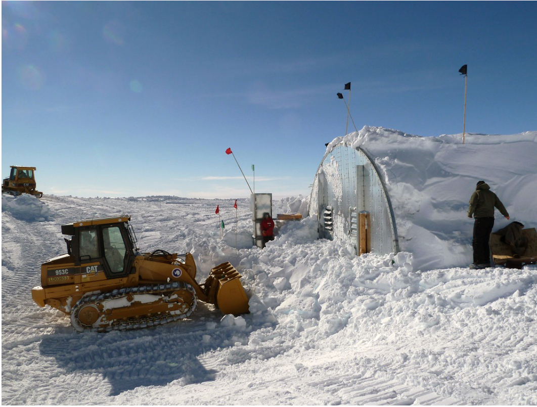
Digging out the doors to the drilling and core handling arch at the beginning of the field season. Photo: Kristina Slawny
